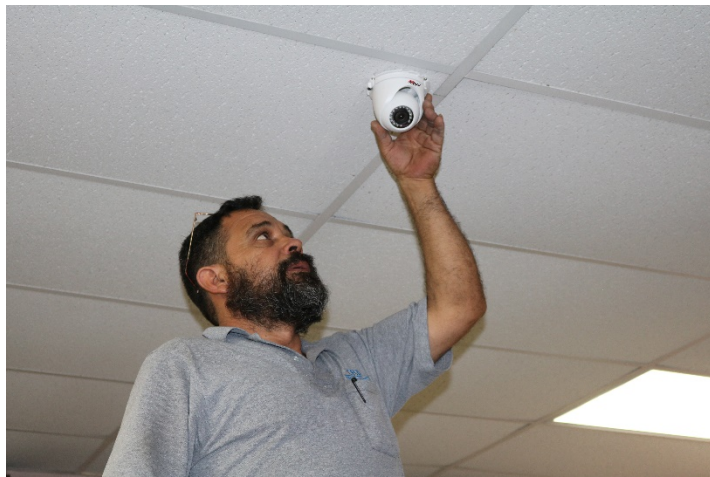
CRB technician Martin Granados installs Dahua IP mini dome cameras
